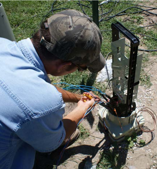
Chris Basgall, Nex-Tech engineering technician, splices fiberoptic cable in rural Trego County.
